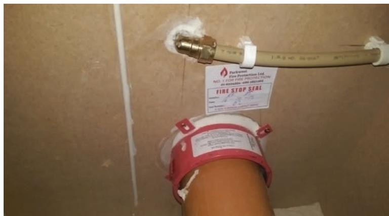
give rise to an opening that will allow significant fire and smoke spread. Proprietary fire seals, including externally-mounted collars, or fire-resisting enclosures, are used in new buildings and could be used to address this problem in older blocks. However, the difficulties of retrofitting such seals in an occupied block of flats may mean that it will only be practicable to undertake this on a long term basis as and when flats become vacant.
