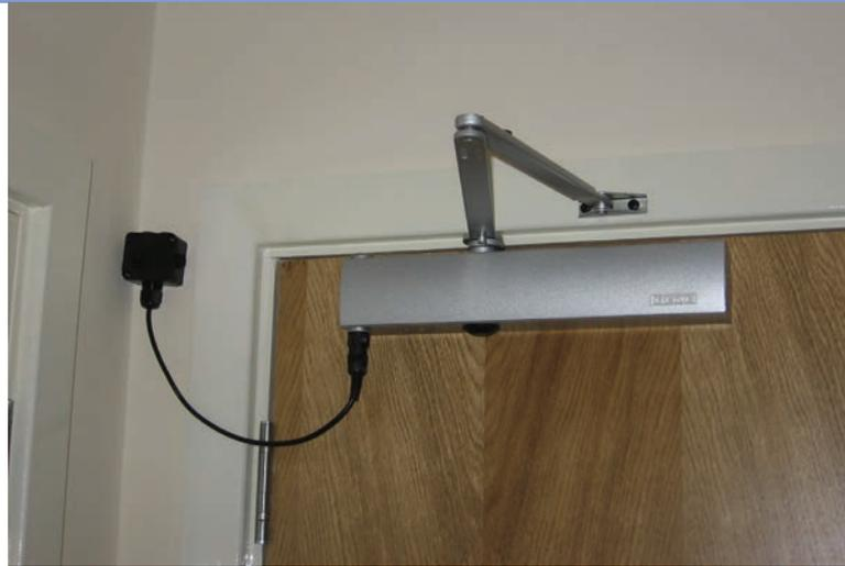
77.85 The fitting of any hold-open devices or swing-free door closers in sheltered and extra care housing can only be permitted if there is a suitable fire detection and alarm system fitted throughout the areas where these devices are used. Recommendations for the fire detection are given in BS 7273-4.
