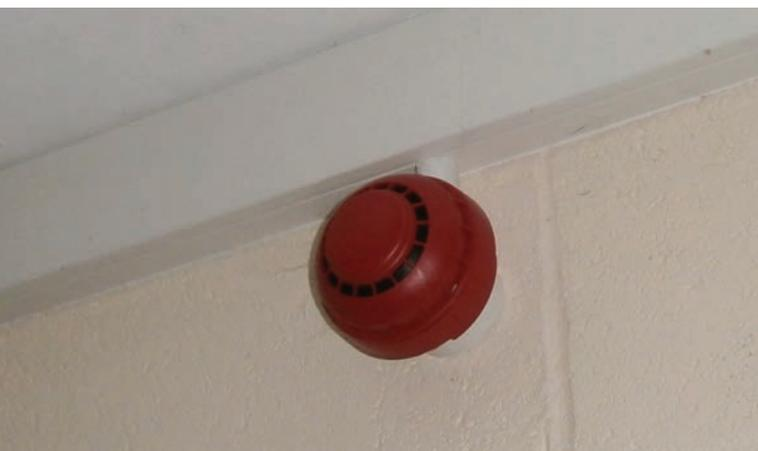
83.9 In areas other than bedrooms, the sound pressure level of the fire alarm system need not be as high as found in commercial premises; typically, a sound pressure level of 55dB(A) will be sufficient. However, care should be taken to ensure that the sound pressure level, frequency and other characteristics of alarm sounders
