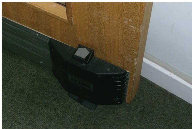
fire alarm system and the failure of the power supply. Other than in the case of doors to protected stairways, acoustically-actuated hold-open devices are acceptable. BS 7273-4 provides recommendations for the design, installation, commissioning and maintenance of door release mechanisms.
